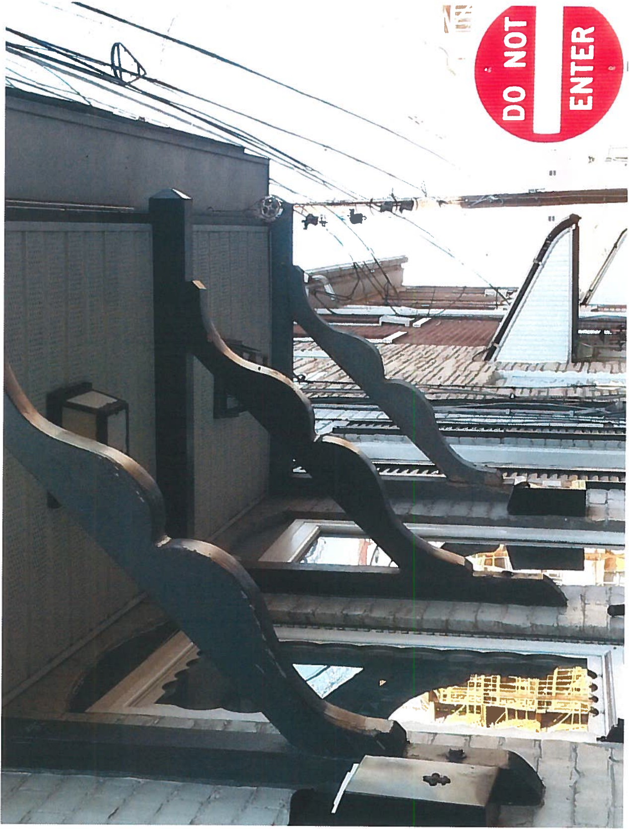
Entry Overhang Structure- side view
